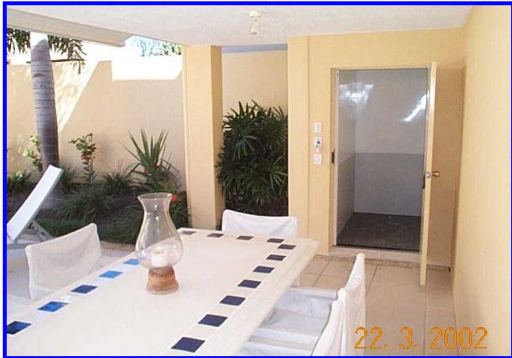
Internal Lift with External grade doors
