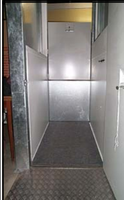
◆ VIEW OF THE LIFT CAR FROM THE LOWER LEVEL
