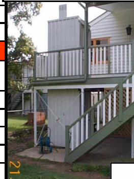
◆ MONOCLAD SHEETING TO OUTSIDE OF TOWER
