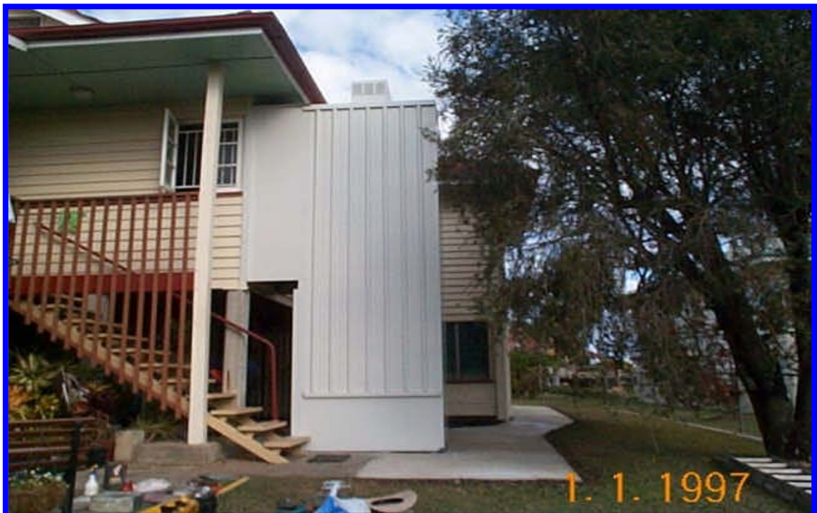
External Wall Penetration
