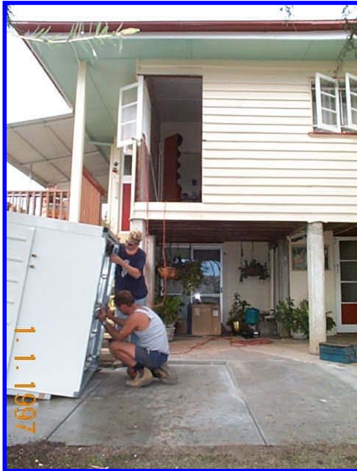
External Wall Penetration Under Construction
