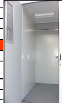
◆ CAR INTERNAL VIEW ◆ CAR MOUNTED EMERGENCY TIMER LIGHT
